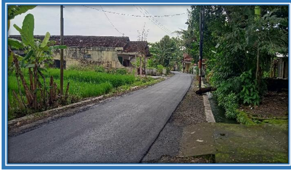
Rehab Jalan Aspal
